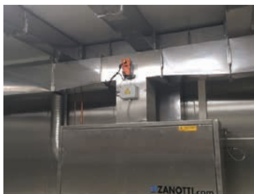
Air distribution system with zinc-coated steel ducts, complete with cones, and adjustable suction devices
