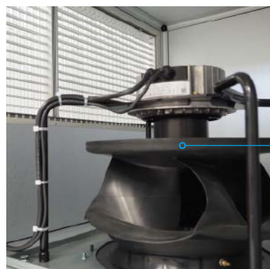
EC fan with speed control
