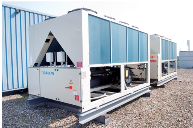
Air cooled chiller installation
