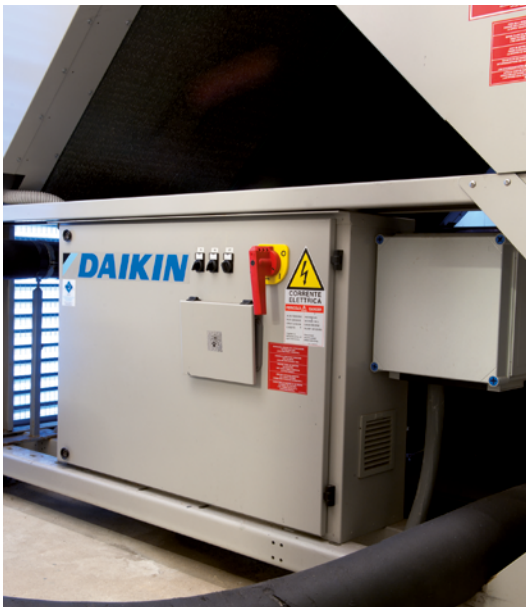
Air cooled chiller installation
