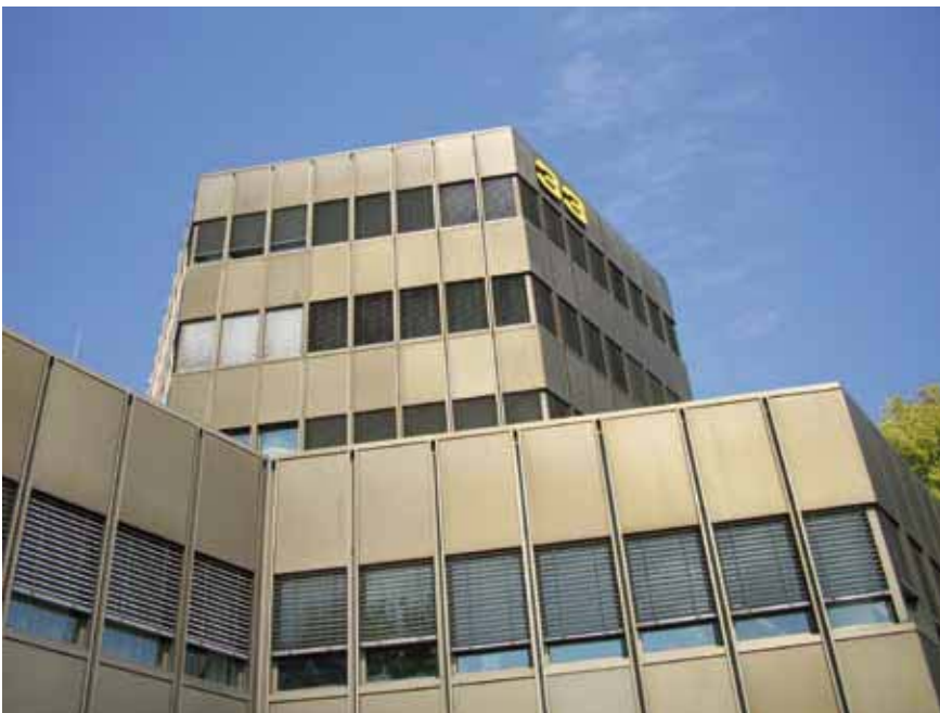
→ Siemens Bacon Building in Vienna: Efficient chiller application using free cooling option.
